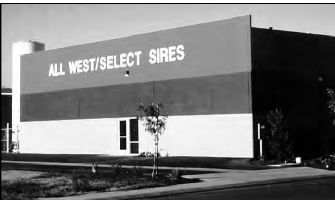
New Turlock Facility nearing completion in 1995
