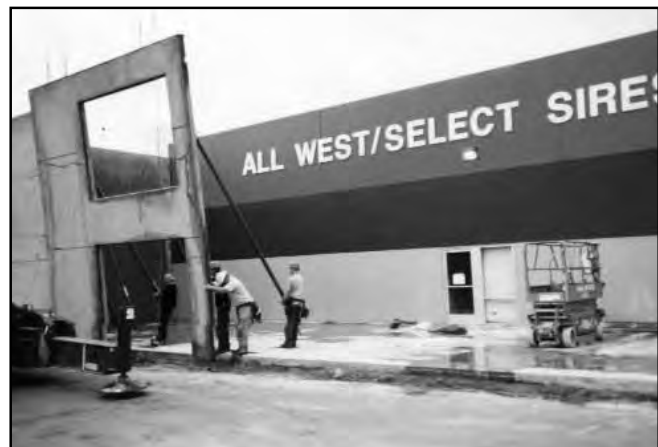
Expansion of office and warehouse facility, Turlock.
